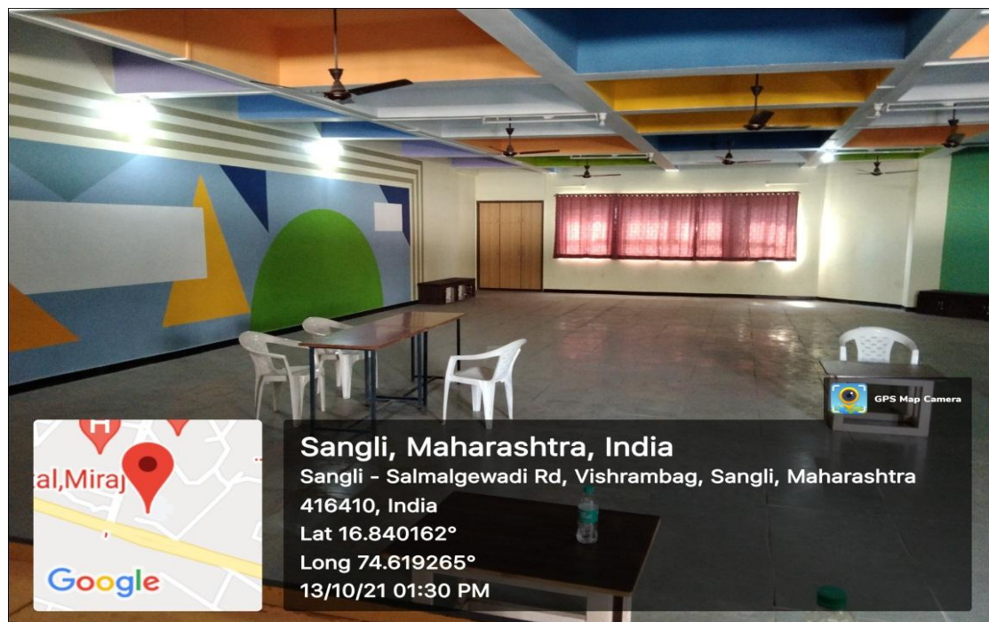
Plate No.19: Replacement of incandescent bulbs by LED bulbs.
