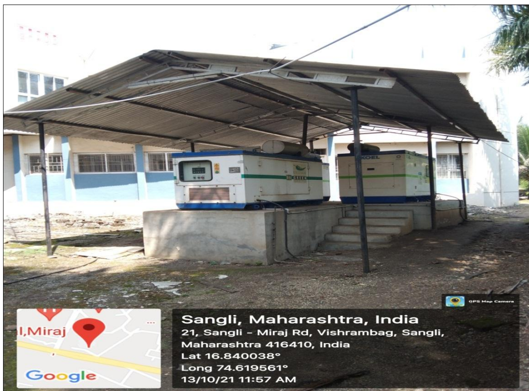
Plate No.17 :Green Power Generator operated on Diesel at VPIMSR.
