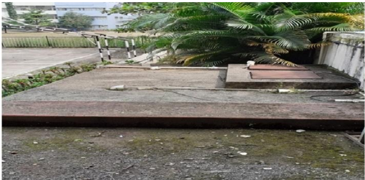
Plate No. 24 A: Rain water collection and storage at CSIBER Institute.
